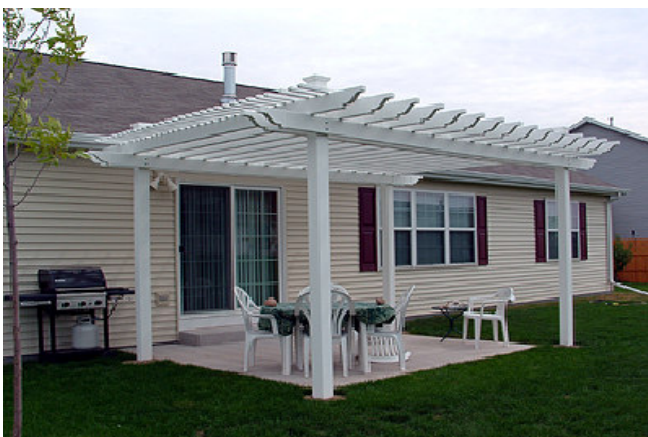
Approximately 12' x 16' pergola Free standing 1 1/2" x 5 1/2" beams and joists 1 1/2" x 1 1/2" laths
