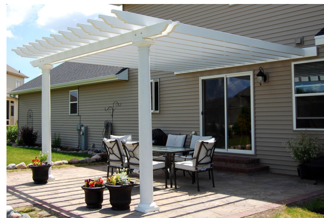
Approximately 16' x 16' pergola Attached to house 2" x 6" beams and joists Round fiberglass columns
