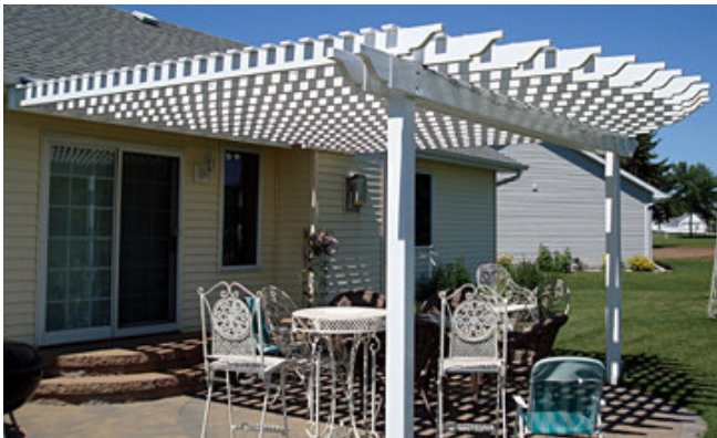
Approximately 16' x 16' pergola Attached to house 2" x 8" beams 2" x 6" joists Joists have been cut to give a rounded look 7/8" x 3" laths
