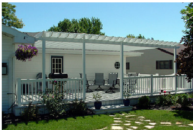
Approximately 14' x 25' pergola Attached to house and mounted to deck 2" x 6" beams 1 1/2" x 5 1/2" joists 7/8" x 3" laths
